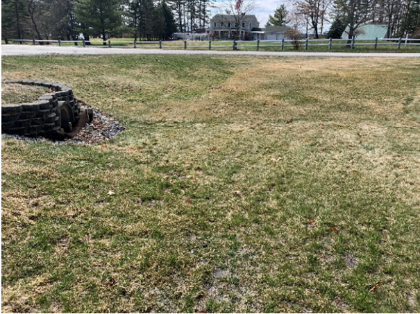
29 Gundalow - 1 (Drainage Area)
