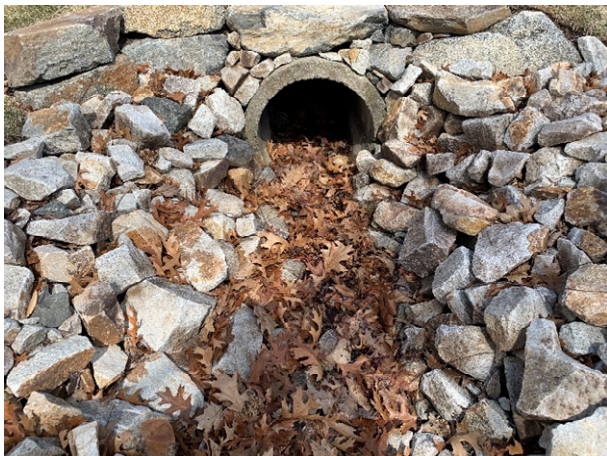
64 Gundalow - 1 (Drainage Course)
